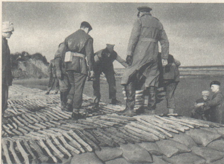
At Mablethorpe, troops strengthen their sandbag sea-wall with fencing.
