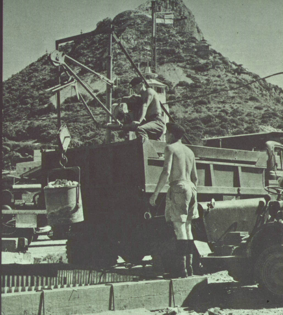
Bringing up spoil from the Windmill Hill shaft (see pictures on previous pages). Sapper Elbrows watches as Sapper Perry works the hoist.
