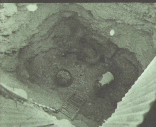
◀ Far left: A Sapper climbs the shaft from Harley Street tunnel while directly above him (left) two more men "muck out" the descending shaft.
