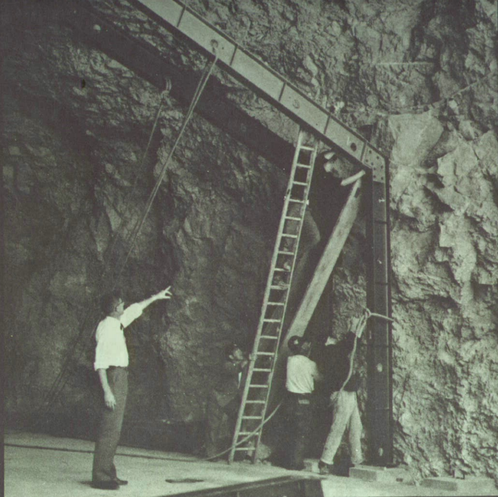
▲ Supervised by Staff-Sergeant C Brynolf, Royal Engineers, civilian workers erect the southern (Europa) portal of the Keightley's Way tunnel.
