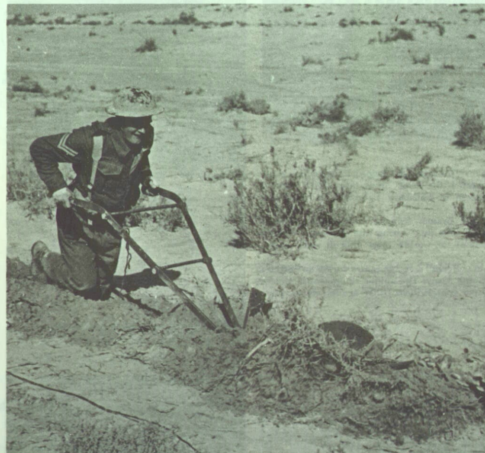
Ploughing a channel for a land line in North Africa in World War Two. The signaller's job has always been much more than tapping a key or lifting a telephone. Later the plough was mechanised.
