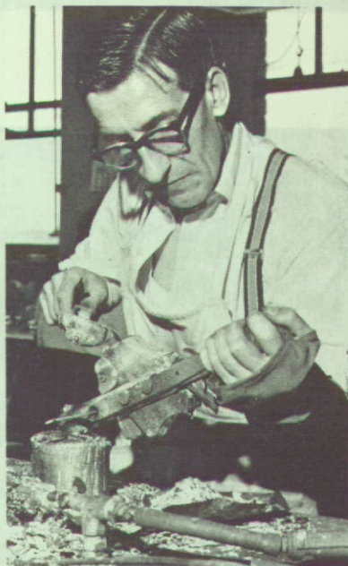
Left: Mr Thomas Barke "slush" moulding—the hand process of moulding hollow figures on which the firm built up its trade. Above: Mr Denis Britain, managing director, with the newest (an electrically operated elevator) and oldest (Life Guard) models. Below: Hand-trimming newly cast metal.
