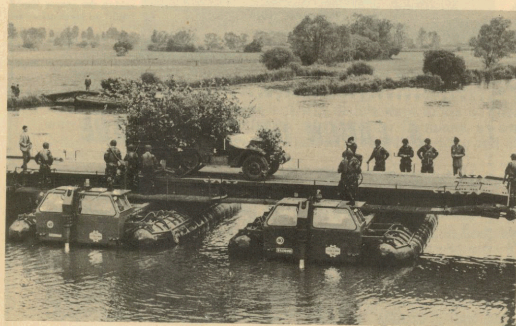
A camouflaged half-track crossing a Gillois bridge.
