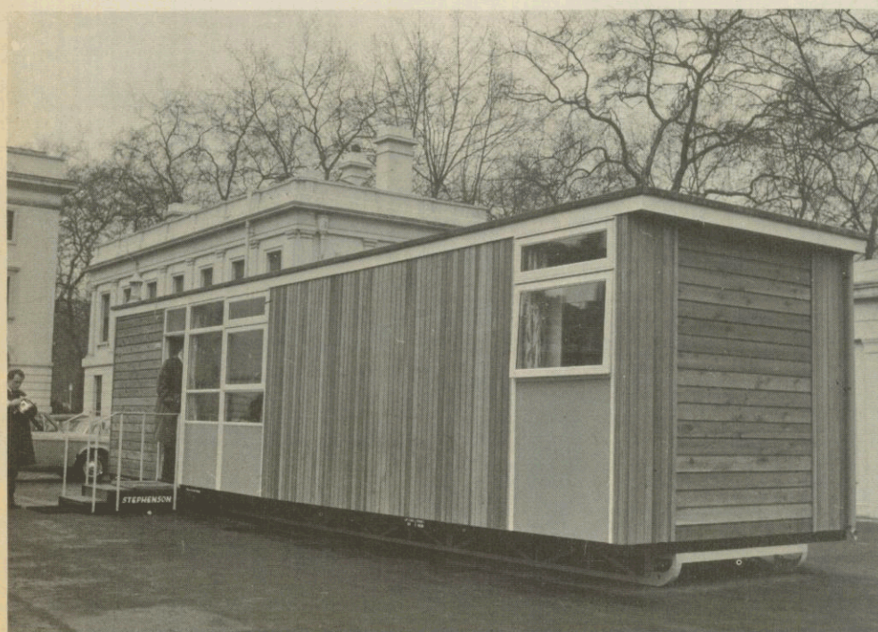
One of the mobile homes on show to the Press at Wellington Barracks, London. The rounded ends of the "ski" chassis enable the homes to be slid into place.
