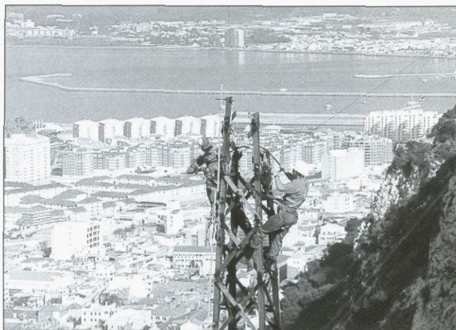
High there: Cpl McBride and Spr Forbes dismantle an old wooden communications mast at Alameda
