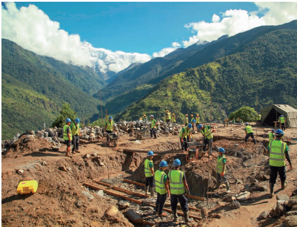
Rugged rebuild: Sappers construct a quake-resistant school
