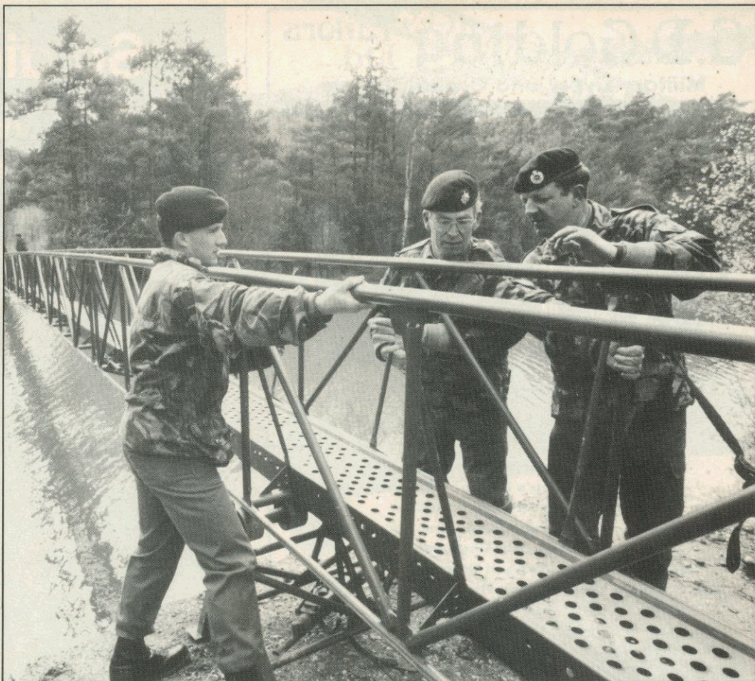
TA assault pioneers clip the last section of Infantry Assault Bridge into place on Hawley Lake
