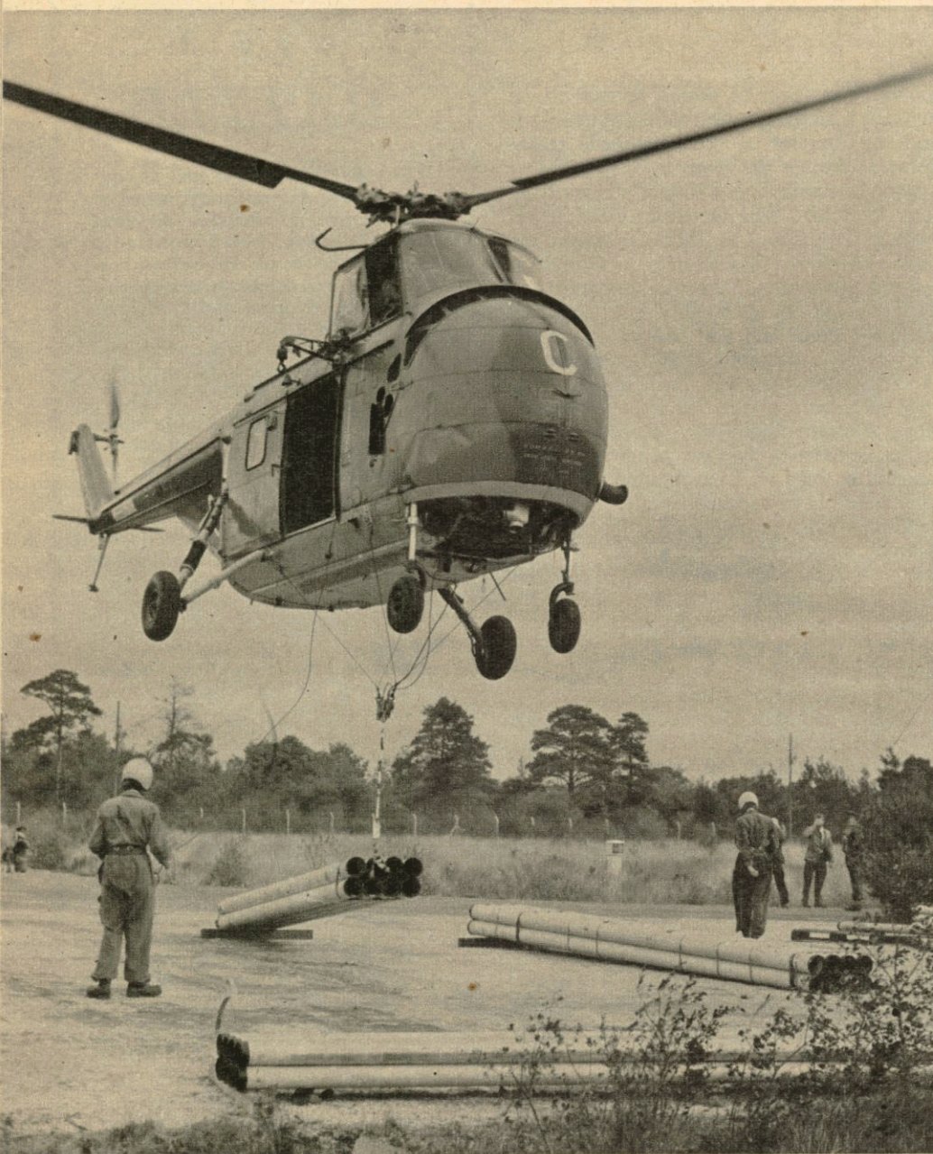
A Whirlwind helicopter hooks up a bundle of eight six-inch alloy pipes—pre-packaged by the Army Airtransport Training and Development Centre—and whisks them away to the Sapper pipelayers.
