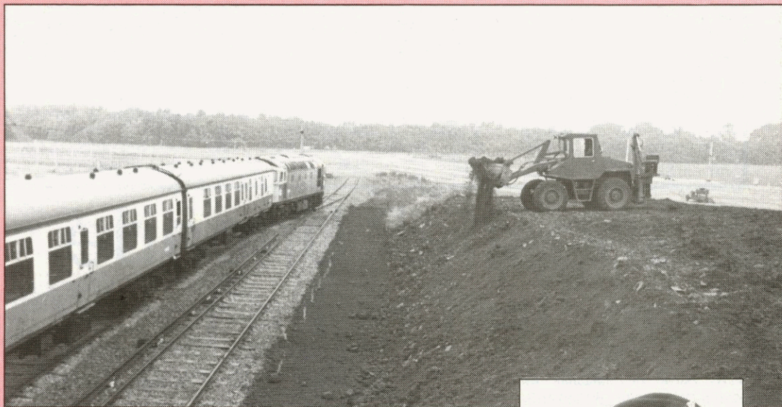
One of the final tasks ... creating a 100-metre long embankment beside the track
