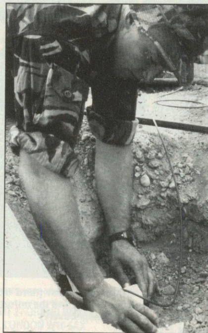
Spr Steven Diplock places a concussion charge in a cavity created using a smaller charge to achieve best effect
