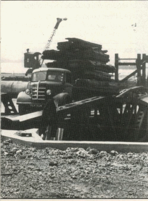
Below – a lorry loaded with much-needed supplies of timber drives ashore over Whale bridging connecting ship and shore at Frog Island
