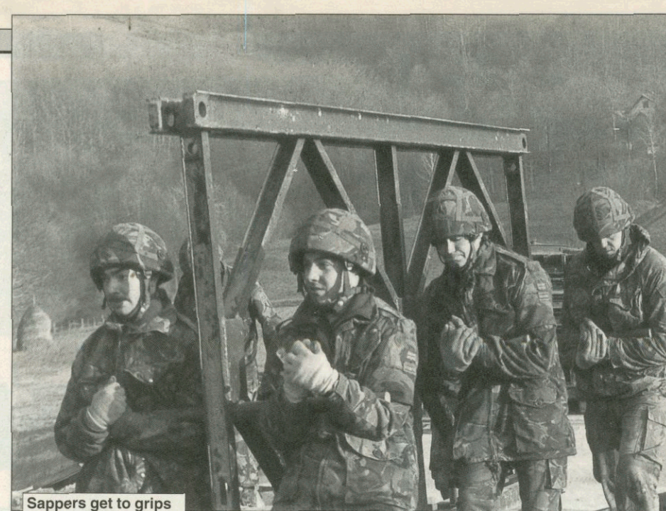
Sappers get to grips with Bailey panels on the Perie bridge site
