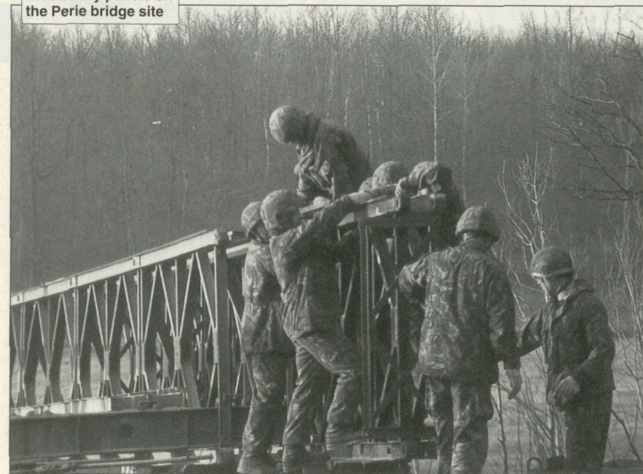
Sappers get to grips with Bailey panels on the Perie bridge site
