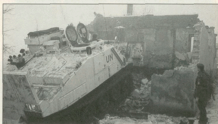
Right – A combat engineer tractor (CET) of Combat Support Troop, 11 Fd Sqn, moves in to demolish a ruined building in a clearing programme for a local community at Vitez
