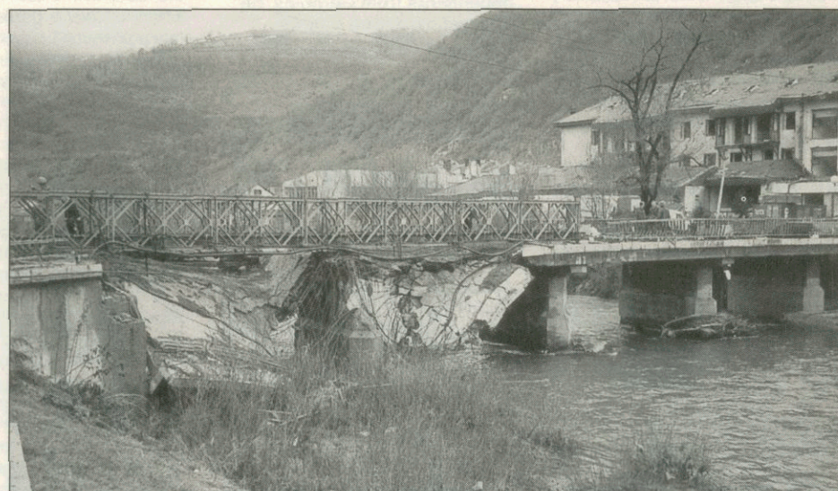
Above – A Serb-constructed Bailey bridge at Donji Vakuf before it was upgraded by 5 Fd Sqn
