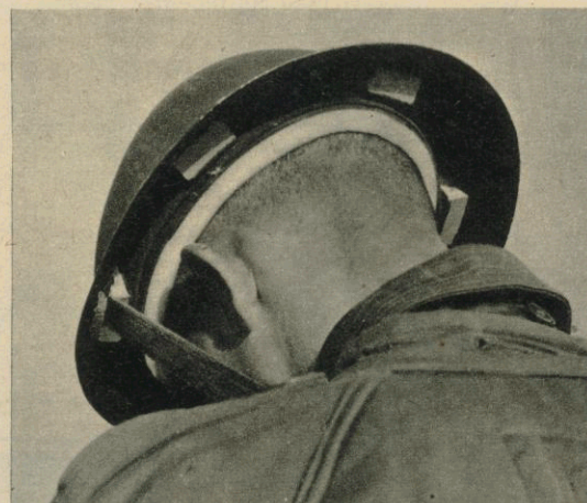
Steel helmets will have a foam rubber liner over which goes a nylon cloth to soak up sweat.
