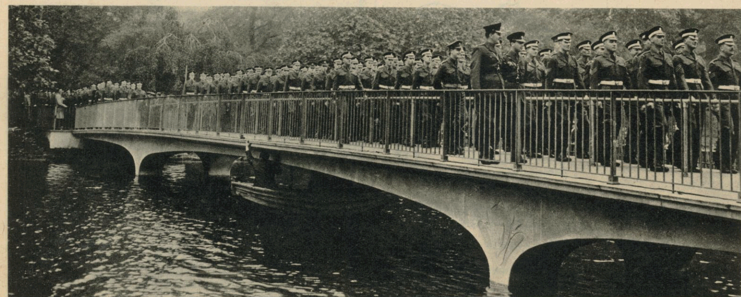
As the Coldstreamers march over the bridge engineers in a row boat measure the stresses.
