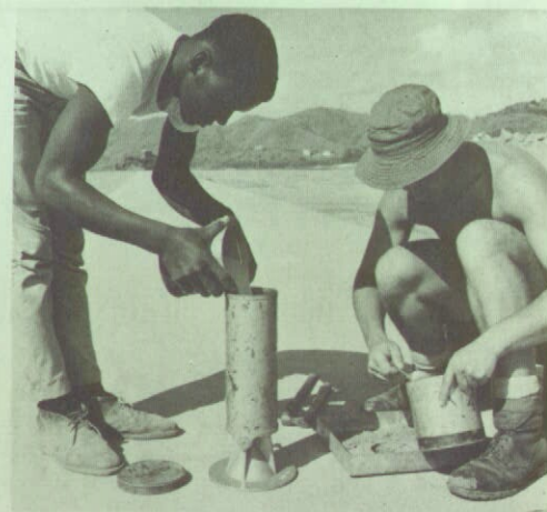
Above: Quality control. A sapper and a locally employed labourer check a sample. If wrongly laid or compacted the runway could crack. The capital cost of the airfield is £216,000—to be borne by the Ministry of Overseas Development.
