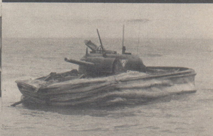
The old way: Britain's swimming tanks, as used in World War Two, elevated their "skirts," as in picture on left, and thus became floatable. The skirts were dropped for landing.
