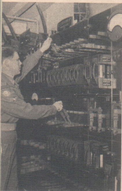
The switchboard of a fort. Two 80 horse-power engines provide fuel and power.
