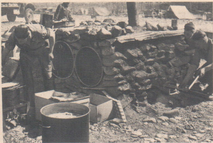
This business-like oven was made by Serjeant R. Ball, Army Catering Corps, from six 40-gallon petrol drums, mud and rocks. It fed 200 men of the Argyll and Sutherland Highlanders.
