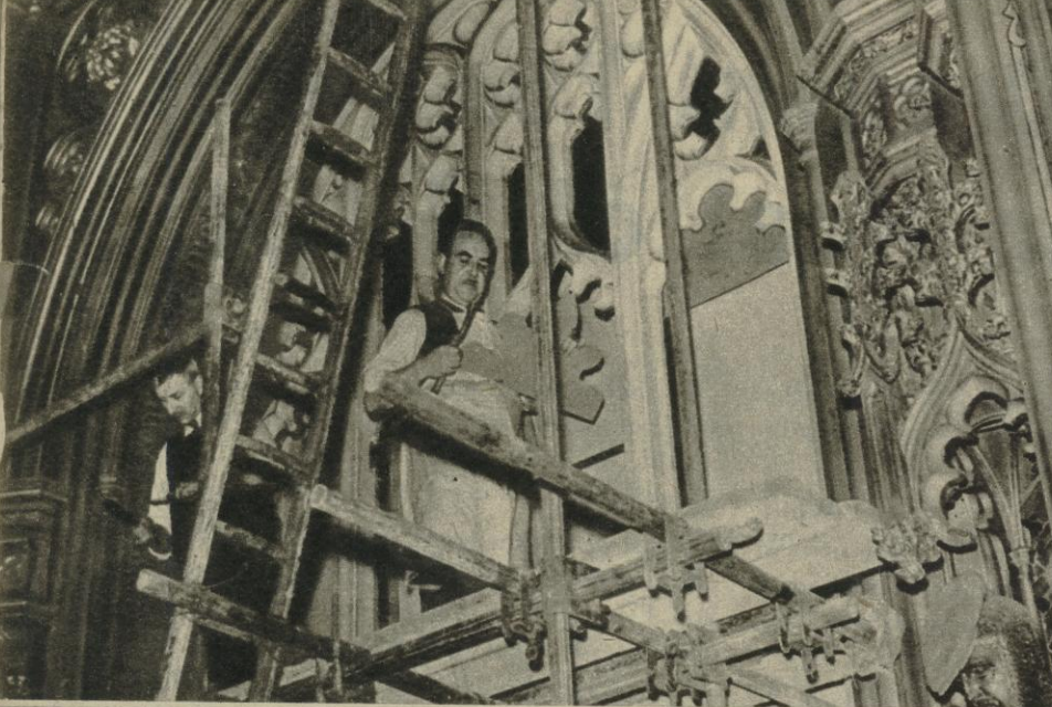
A workman prepares a template for fitting glass to windows of the Lords' Chamber, used by the House of Commons since the 1941 blitz.
