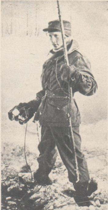
**Left:** Using an ice saw. A preliminary hole is drilled with an auger. The saw will cut through ice a yard thick.
