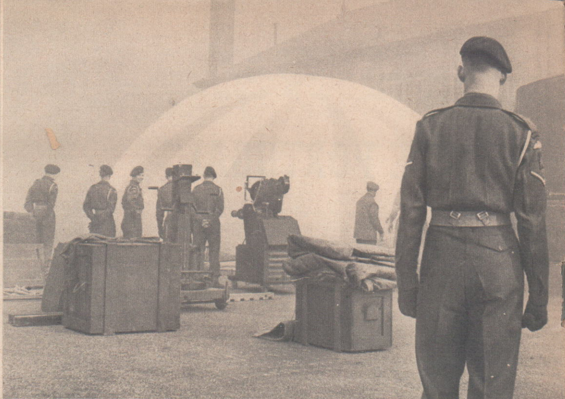
Going up... The Portobel will stand high winds, for the dome is lashed to a base of concrete sections bolted together.
