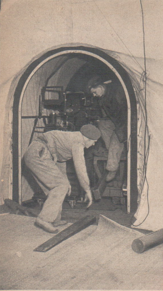
The airlock door is big: it has to be, for through it comes all the training apparatus after the dome has been inflated.
