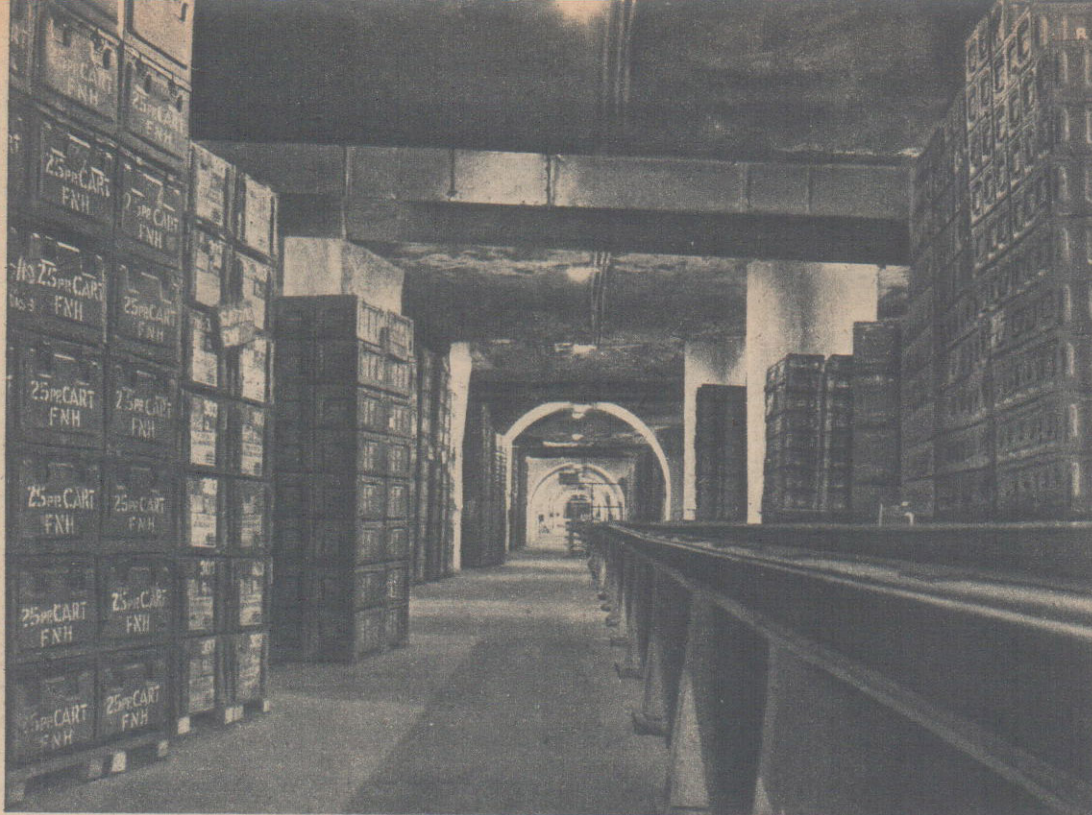
An underground ammunition district, showing the electric conveyor belt running through the centre of the tunnel. There are ten districts in the subterranean depot.
