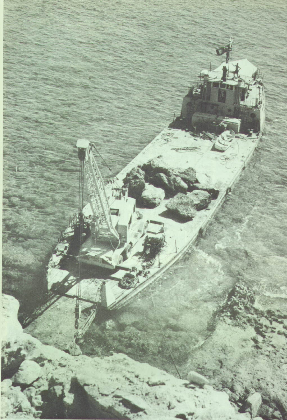
Left: Another huge rock for the mole is man-handled by a heavy crane at one of the quarries.
