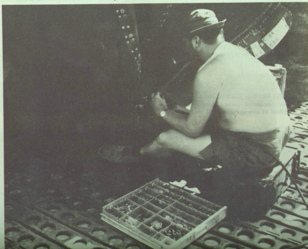
Naval air mechanic David Reynolds carries out repairs on the fabric skirt of an SRN5.
