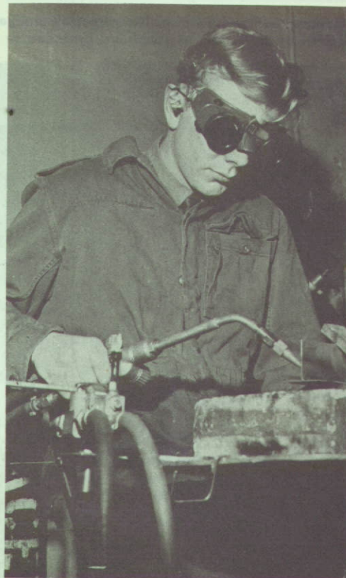
Welding course students learn electric welding (above) and gas welding (below). Subsequently they move on to a government training centre.
