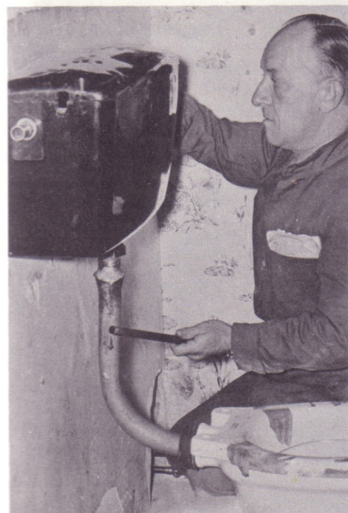
Below: Installing a toilet suite is another art taught on the plumbing/central heating course.
