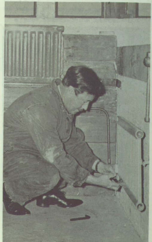
Above: Reassembling an engine on the course for motor mechanics. Below: Fixing a central heating radiator—many men go straight to heating firms.
