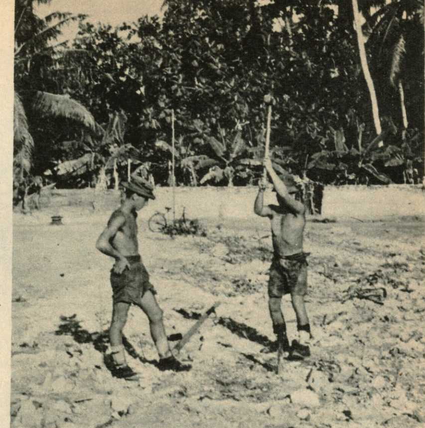
Above, L/Cpl Hughes and Sgmn Smith using hammer and jumper during the erection of a temporary telephone line. Overhead lines fought a losing battle against mobile cranes.
