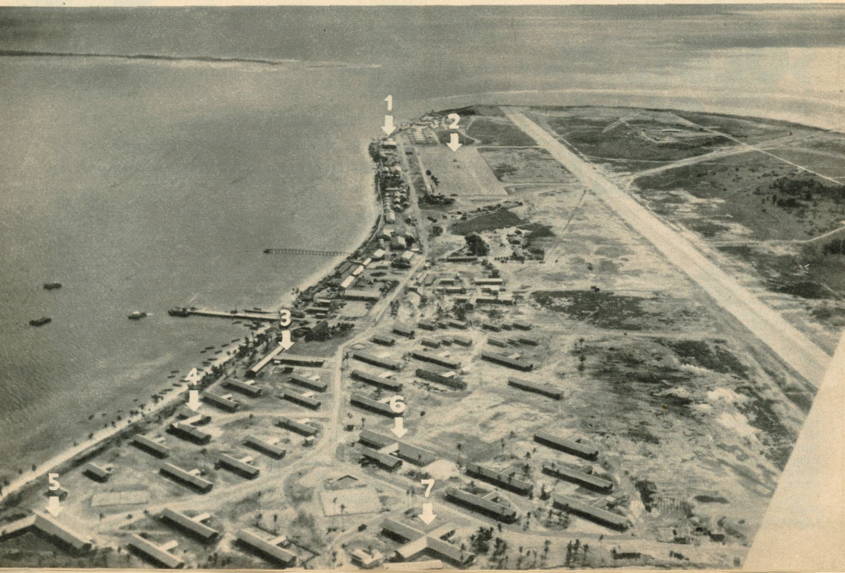
This aerial view of Gan shows part of the new runway, sweeping diagonally across the whole island. Left are the new prefabricated buildings which accommodate the soldiers and 400 airmen on Gan, and the jetties for unloading supplies. Picture key: 1, Cinema; 2, Hard standing for aircraft; 3, Hospital; 4, Sergeants' mess; 5, Officers' mess; 6, Dining hall and transit; 7, NAAFI building.
