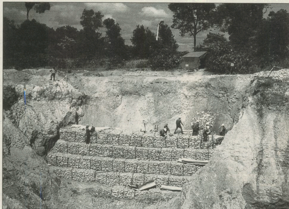
Above – Five rows complete, four to go: the wall which C Troop had to build, to stop the range road sliding away
