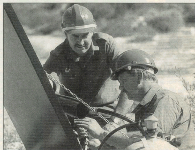
BT Stone training designer Lee Featherstone (right) closes a 50-pair cable joint near the Episkopi base, assisted by Manchester North joiner John Ryan
