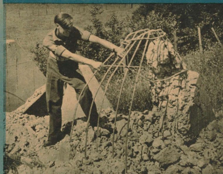
A dragon's tooth is not so difficult to destroy: many of them were shoddy. The explosive applied as in the picture above shatters the concrete from the conical steel framework (See below).
