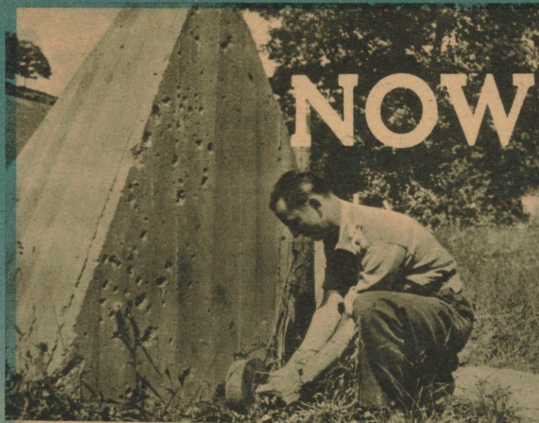
A dragon's tooth is not so difficult to destroy: many of them were shoddy. The explosive applied as in the picture above shatters the concrete from the conical steel framework (See below).
