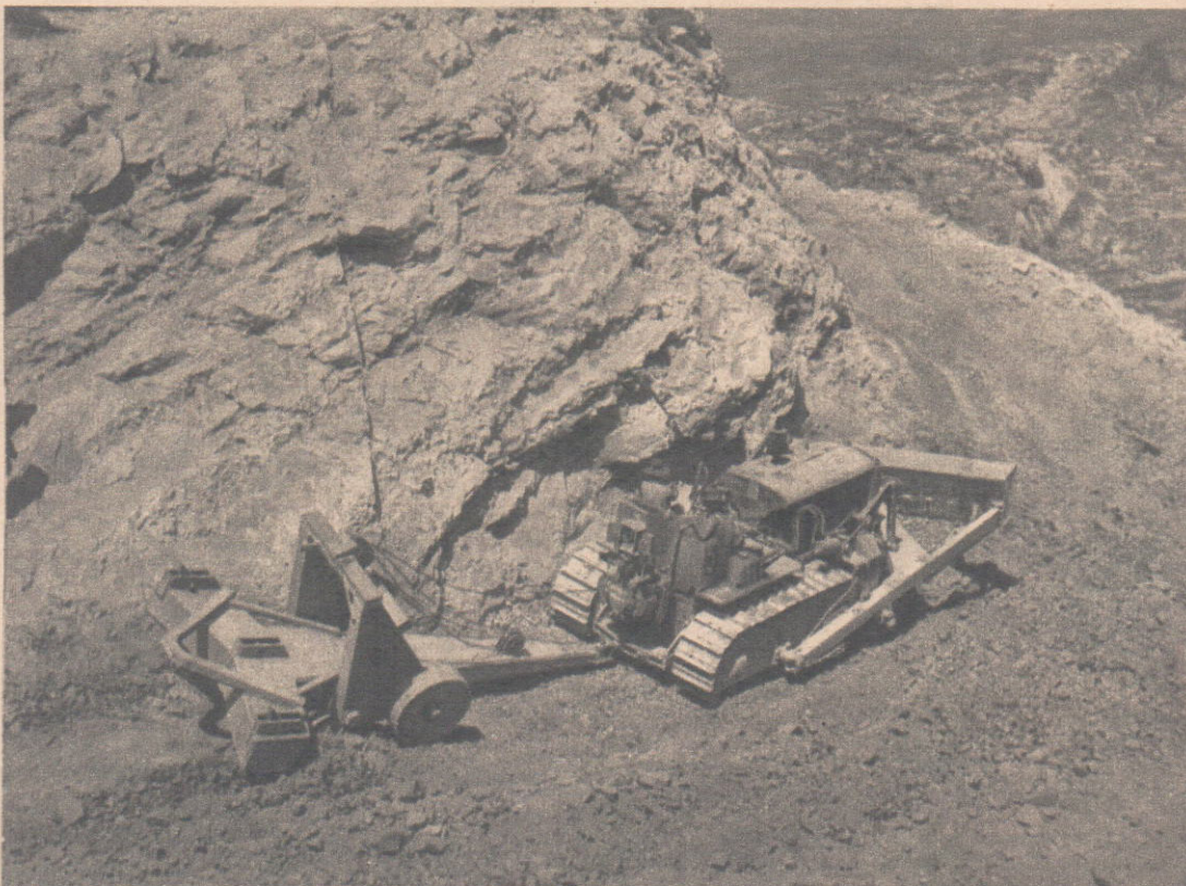
Below: The curious-looking device being towed by a bulldozer is a rooter, a name which explains itself. It is only one of a rich variety of road-building machines which were used by the Allies in World War Two.
