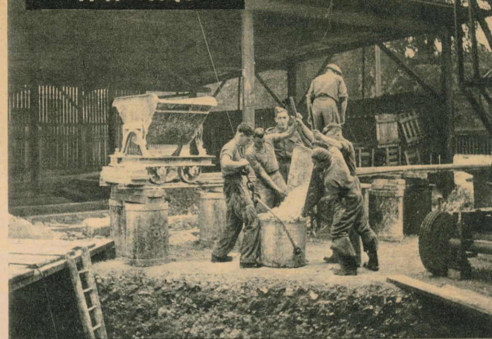
1 Removing the "Woe Waters" bomb at Croydon is a big business. Here is a stage in the excavation work—soil from the shaft being loaded for removal.
