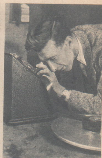
With this instrument a technician examines sound track, judges its density.
