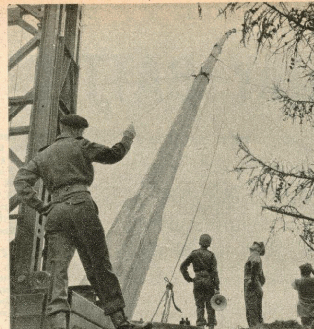
With steel hawsers attached to a 100-ft steel tower, the Sappers haul the new flag pole into position. The pole, 225-ft high, was shaped out of a 300-year-old Douglas fir shipped from British Columbia.
