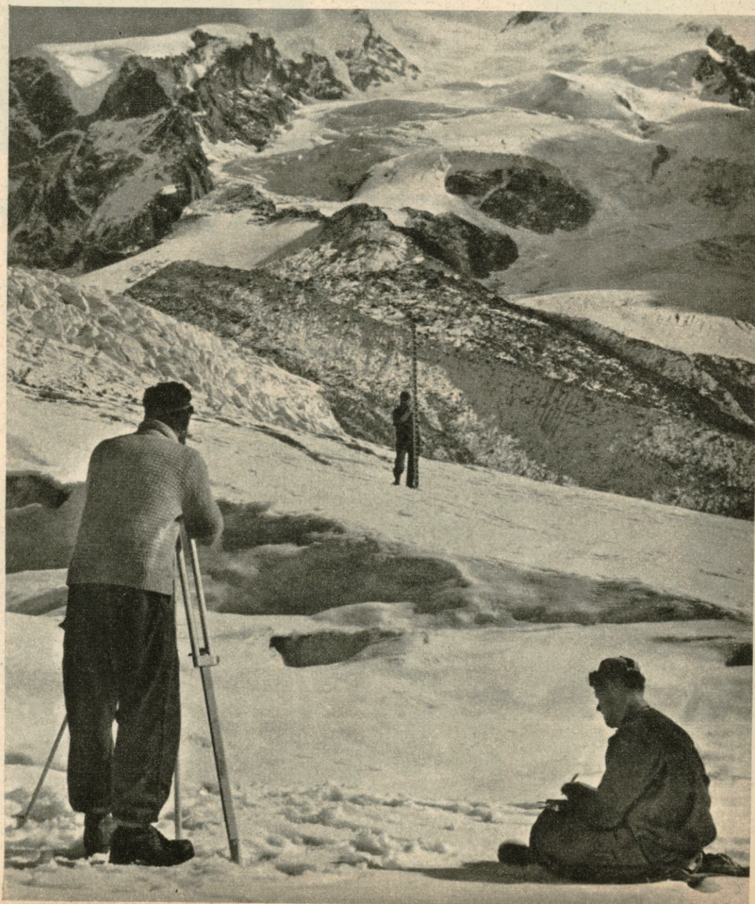
Below: As Lieutenant J. Fullerton takes readings with a theodolite, another Sapper notes the measurements. The team spent ten weeks in the Swiss Alps, living in an Arctic tent.
