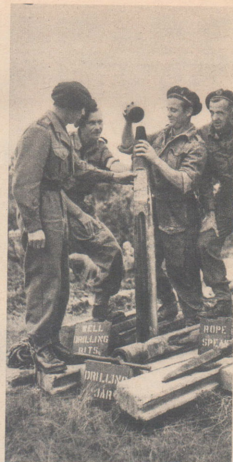
Serjeant-Major Harold Gorbett, Supplementary Reserve (left), shows his men one of the six-inch bits which "percuss" their way down to water. Some bits are of 12-inch diameter.
