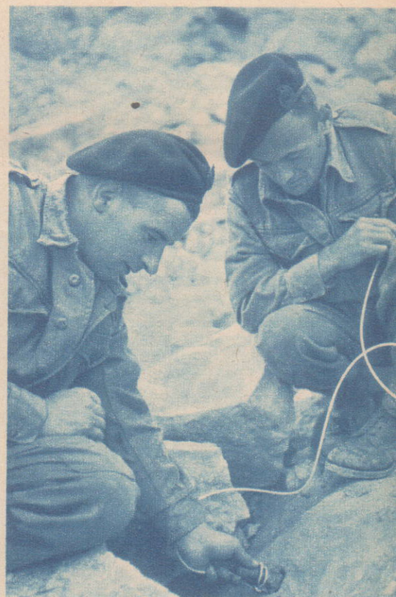
This is their civilian job: two quarrymen from Wales—Lance-Corporal I. Evans and Sapper W. E. Griffiths—prepare a gelignite charge.
