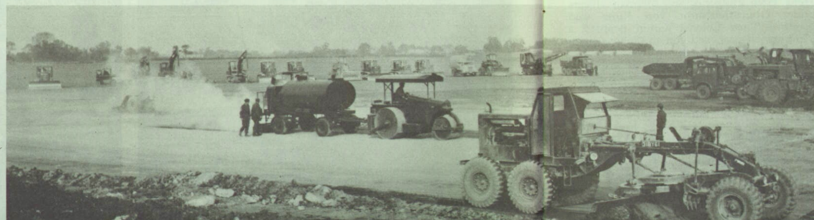
Left: A bitumen distributor trails acrid fumes and smoking pitch. The stationary angle-dozer on the right has been used to level the surface.
