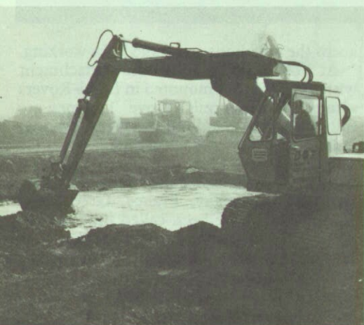
Above: Hydraulic excavator removes soil from a flooded crater. Below: Cyclopean fragments of broken concrete are lifted out in a tractor's bucket. Above right: Crushed granite ballast is nosed into a deep crater by a bulldozer blade.
