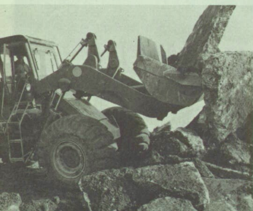
Above: Hydraulic excavator removes soil from a flooded crater. Below: Cyclopean fragments of broken concrete are lifted out in a tractor's bucket. Above right: Crushed granite ballast is nosed into a deep crater by a bulldozer blade.
