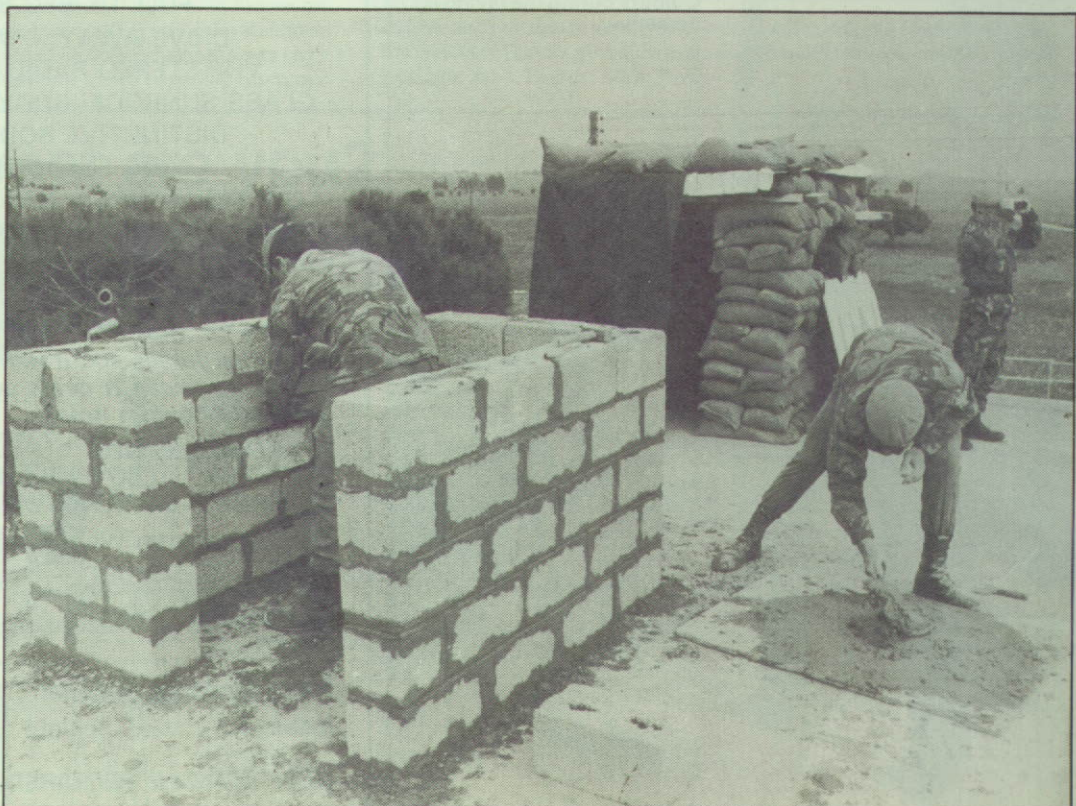
Sappers in support of the DERR rebuild an OP blown down by strong winds
