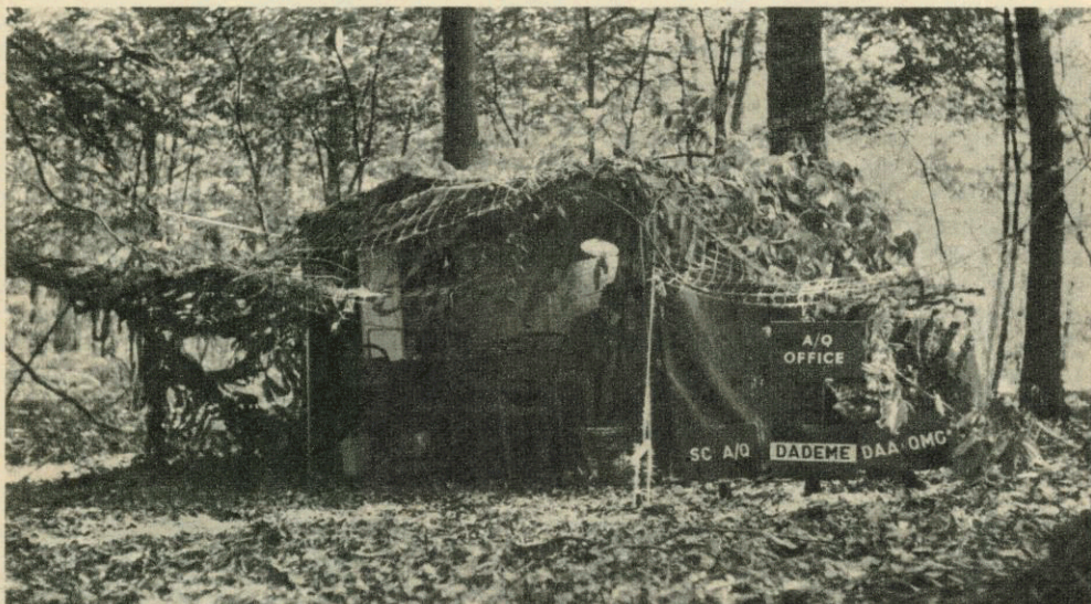
Another product of an inventive mind in the Brigade is this shelter, designed and built by Lieut-Col Douglas Smith, who commands 324 Regiment. Built easily on to the side of a Champ, it is light and portable. As it can be built up on the brick system it is planned to use it for Brigade HQ.
