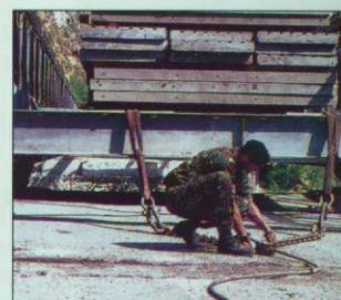
Going: A bridge section is readied for removal
