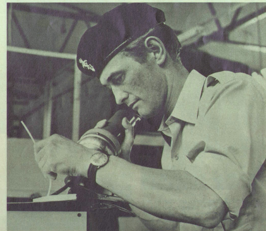
Above: Development work on snorkels by the branch now enables beach armoured recovery vehicles to be effectively used for work in water depths of twelve to fifteen feet.
