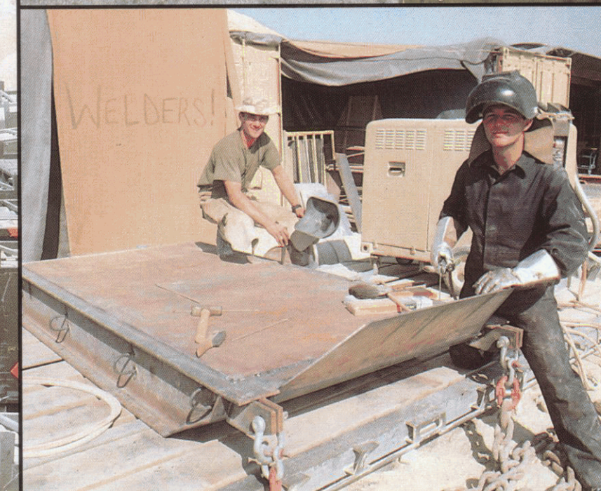
Below: LCpl Jim Hendrickson (left) and welder Cpl Trev Dale of 45 Field Support Squadron RE construct a sledge for towing additional munitions behind armoured vehicles. This is a smaller version of a prototype designed and built in the desert for Challenger
