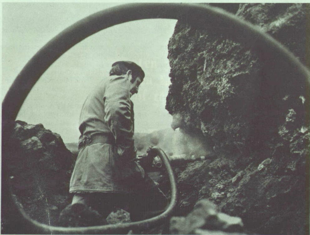
Royal Monmouthshire Royal Engineers prepare an obstinate mass of conglomerate before blasting. Above: The pick and shovel gang may break up some boulders but the drill (below) has a big part.
