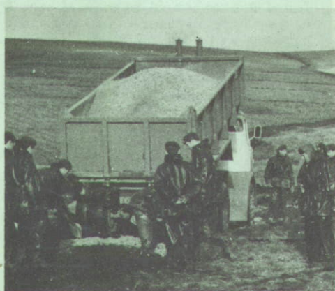
Top of page: Sappers lay pierced steel plating to make a road to carry heavy pumping equipment to Lluest Wen reservoir. Above: Reinforcing the "dual carriageway" with stone from one of the hundreds of heavy lorries that used the road. Below: Colonel Macey at his emergency HQ.
