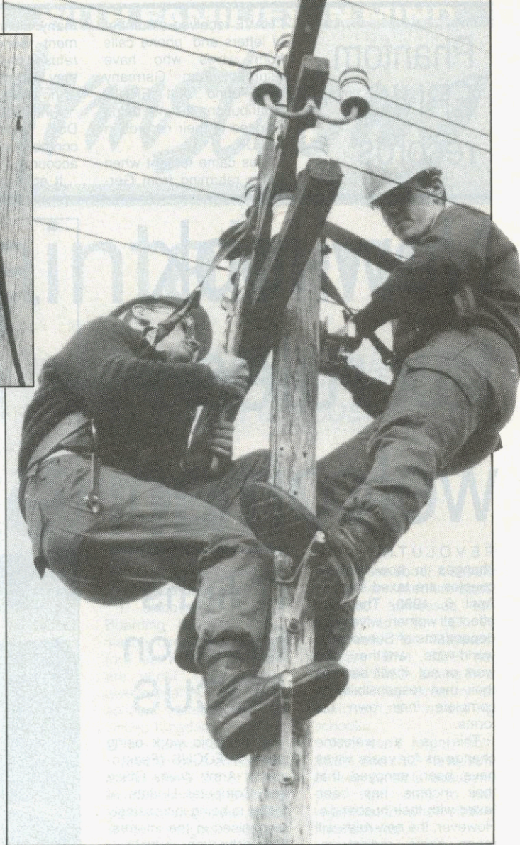
Above - Cpl Colin Burgess terminating a line along the pole route
