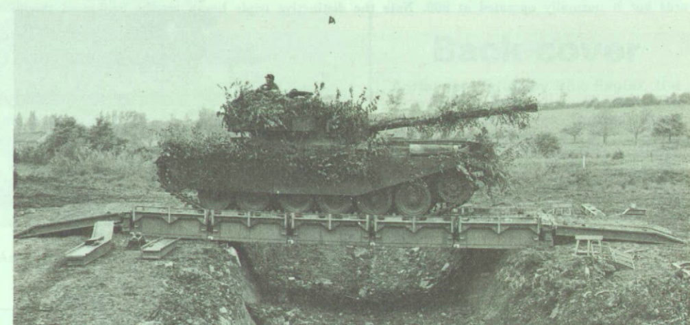
Below: Chieftain crossing the 30-foot single-storey lightweight bridge.
