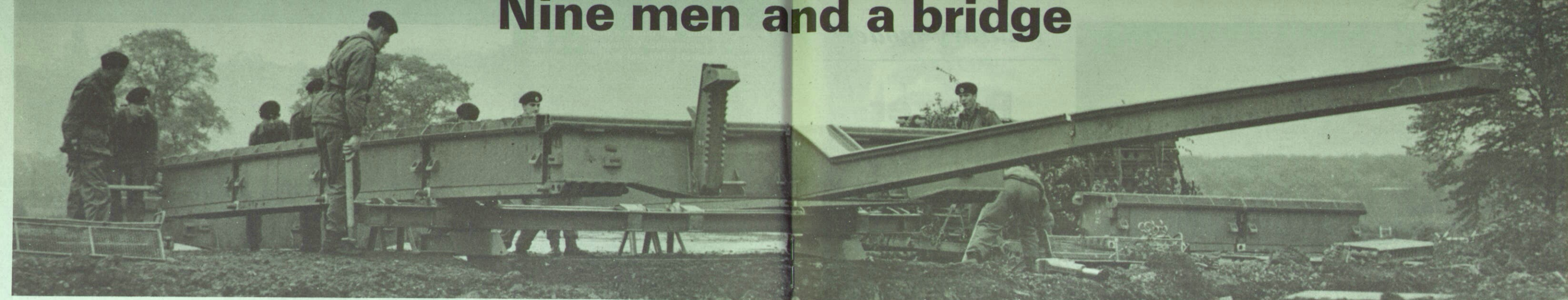
Above: Assembling the bridge—launching nose in position. Below: Unloading the trailers.
