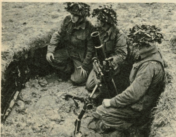
The new 84-mm mortar will replace the 3-in mortar in the next three years. It has a range of over three miles and can fire at the rate of 30 bombs a minute.
