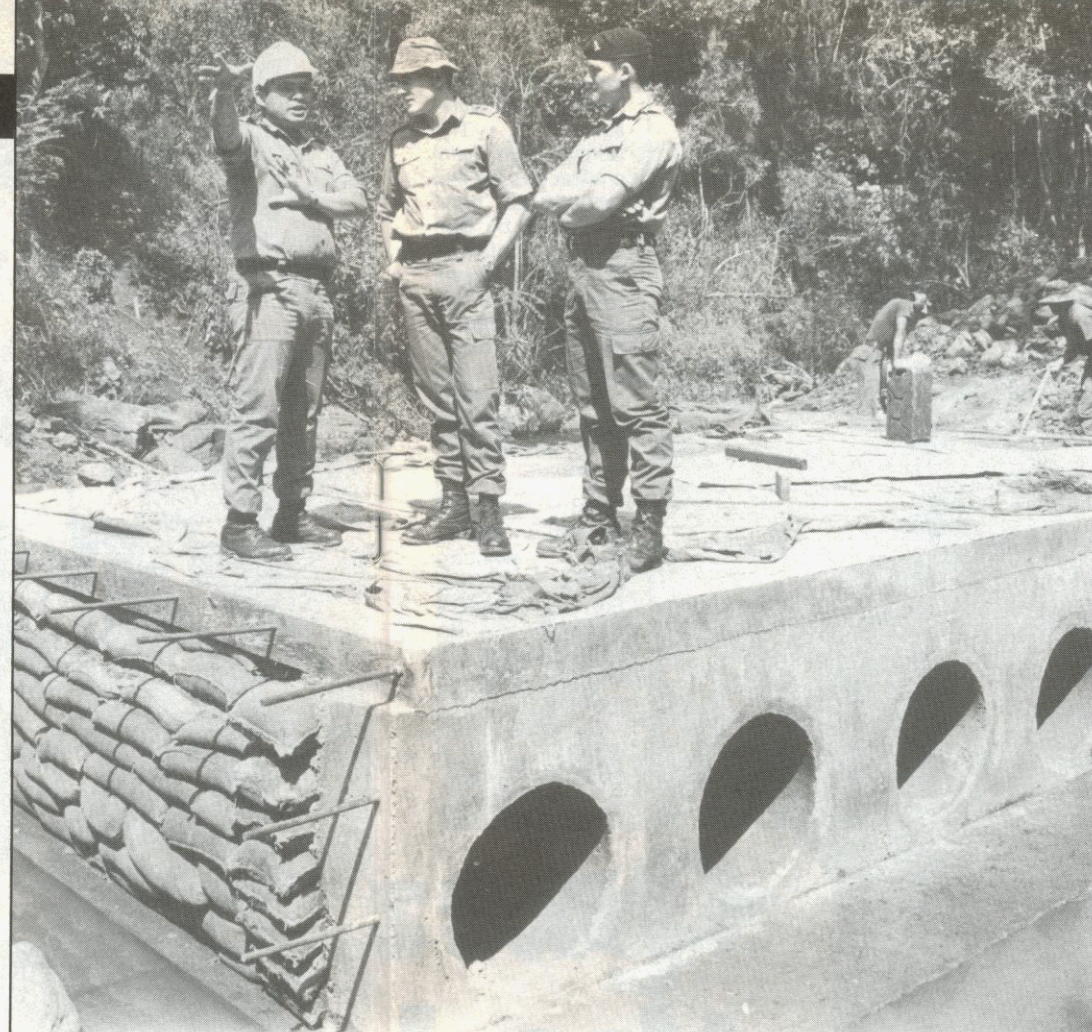
Above - Lt Hom Bahadur Rana shows Lt Piers Vickers and 2nd Lt Mark Crofts how the first half of the Amboni causeway will withstand flash floods
