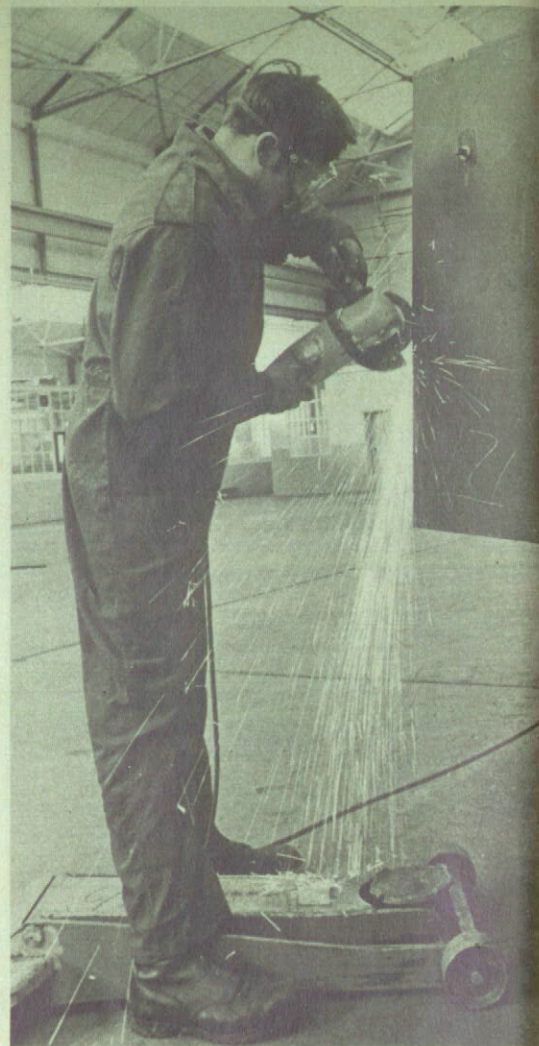
The vehicles' interiors were stripped out to take the new protective armour plating.
