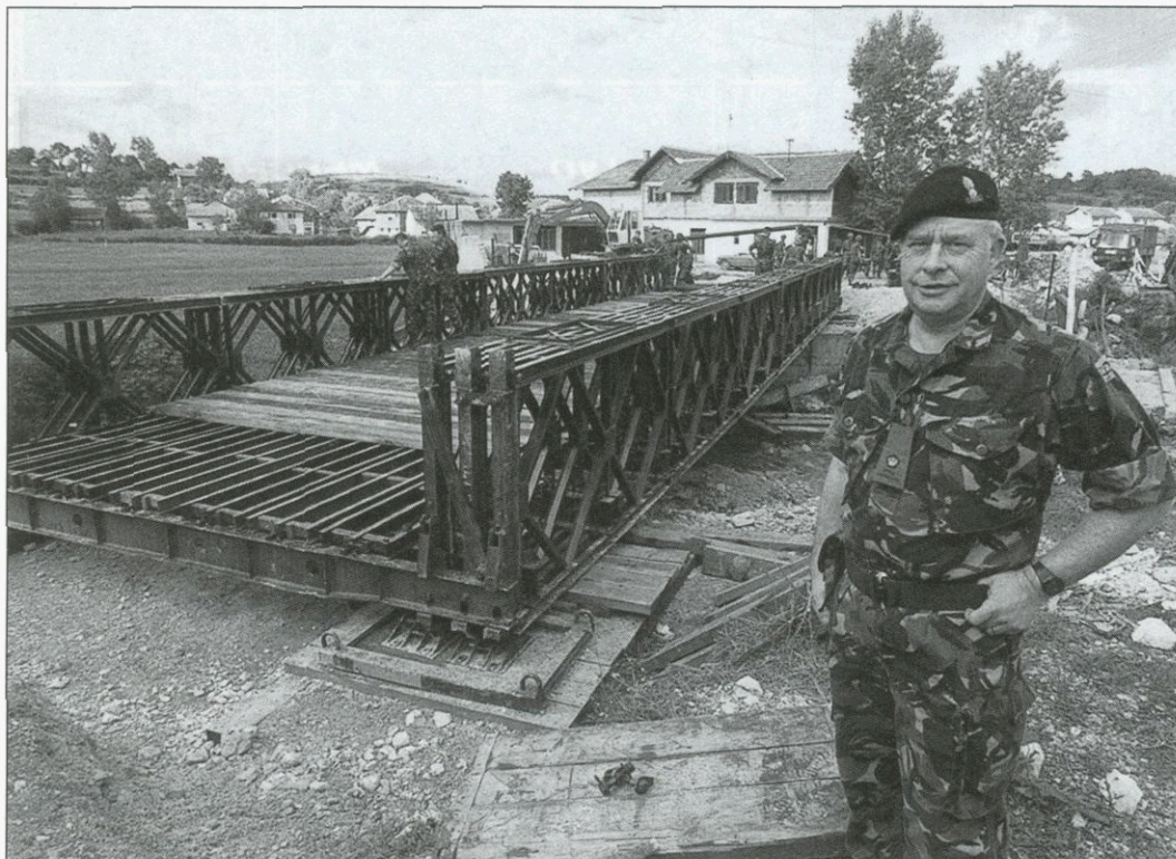
Territorial Army sapper Maj Bill Paynter with the Bailey bridge constructed from redundant stock found by him. Sappers from 3 Armoured Engineer Squadron put up the bridge in time for the Bosnian elections
