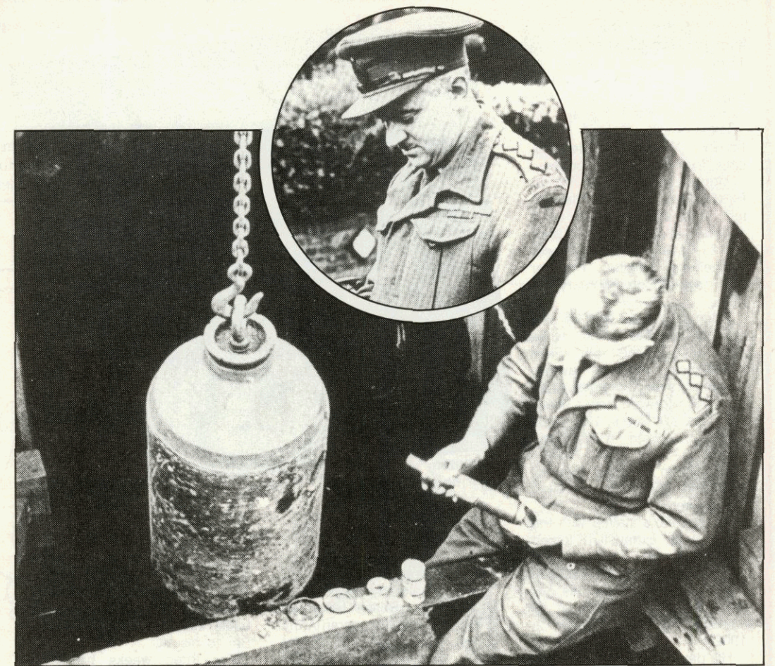
A difficult job for Capt Hunt. It involved a 27ft excavation near the River Lea. Pumps could not cope with incoming water so the bomb was slung, raised to a convenient height and defused. Inset shows Capt Hunt at a less fraught moment.
