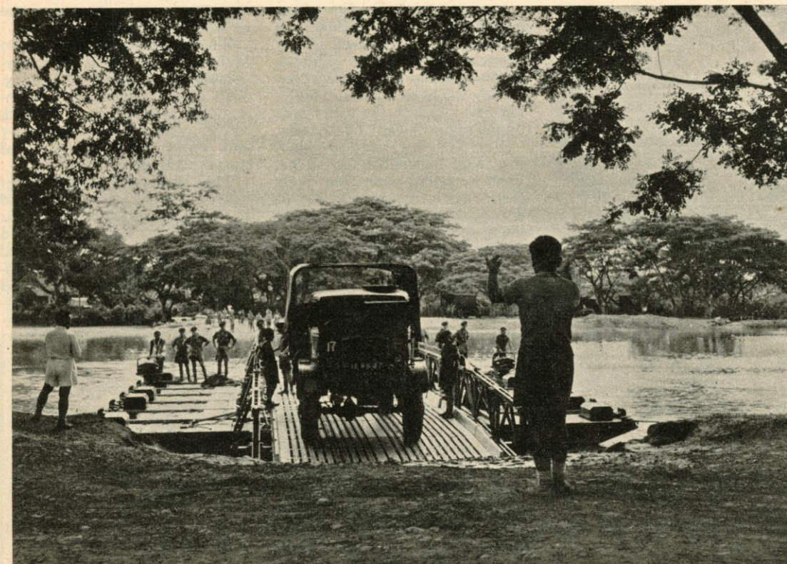
Sappers of 68 Gurkha Field Squadron handing over their tasks after six months in Kota Belud show men of 11 Independent Field Squadron, Royal Engineers, how to operate the light assault floating bridge over the Sungei Tempasuk. A Gurkha signals "come on" to the three-tonner on the ramp.
