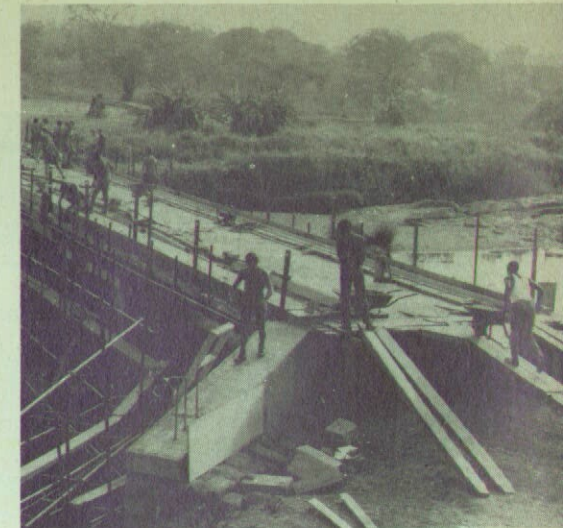
British and Sudanese sappers wheelbarrow cement up wooden planks on the bridge.
